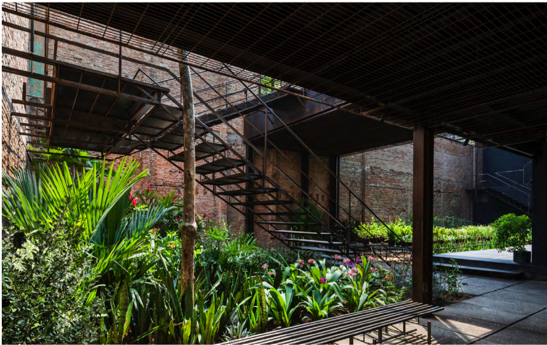
Stairs to pedestrian link (L2)
