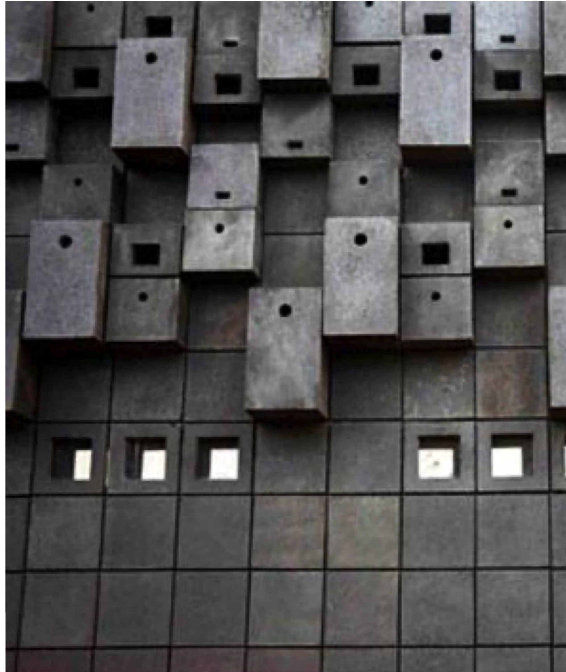
Example of roosting boxes integrated in architectural facade of building
